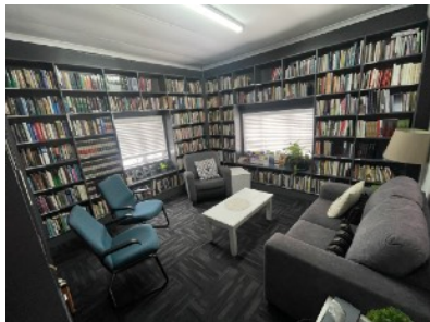
Counseling room/Library floor repaired
