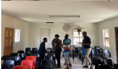
Notice the building improvements in these two photos taken at My Father's House Baptist Church
